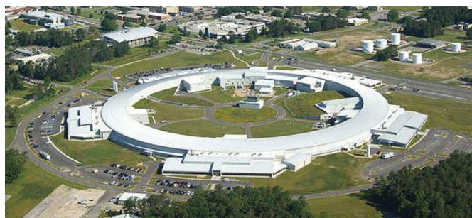
The National Synchrotron Light Source II (NSLS-II) at Brookhaven National Laboratory, for which the US Department of Energy has approved the start of routine operations.
