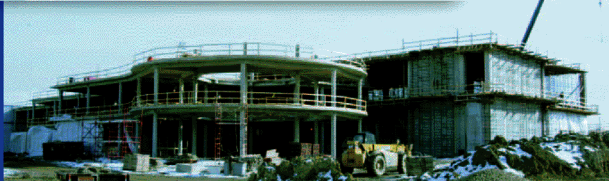
Construction progress at the Argonne CNM, as of 2.2.05.
