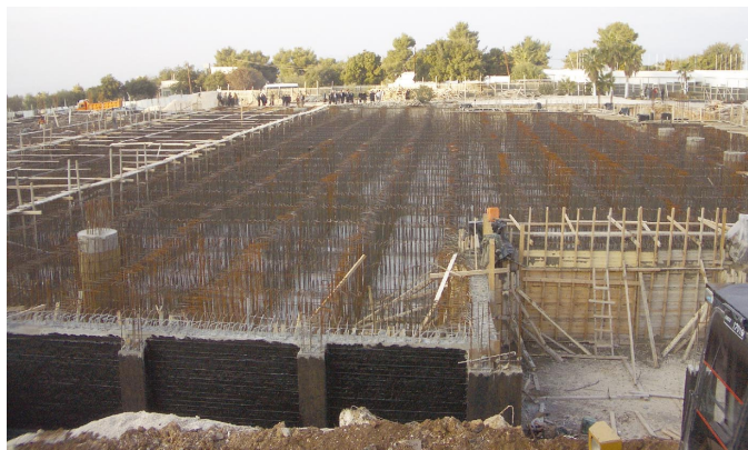
A view of the SESAME building on 14 December 2004.
