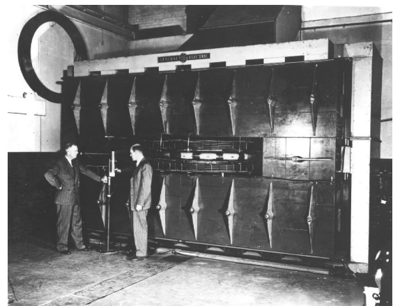
Figure 3 The 100 MeV betatron at the General Electric Research Laboratory with E. Charlton (left) and W. Westendorp.
